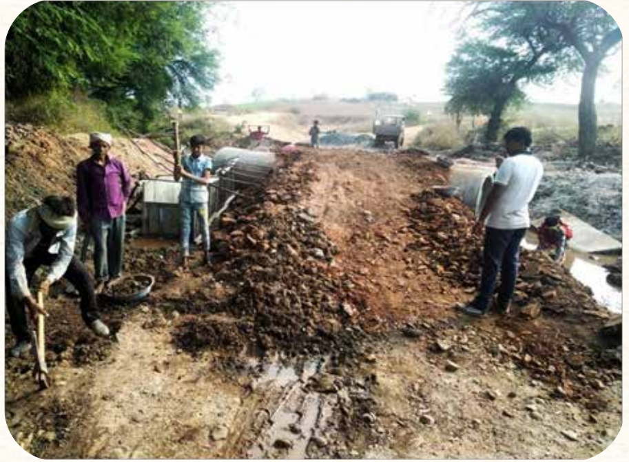
Constructing A Culvert At The Paraspipli Panchayat Under MGNREGA
